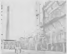
Eastern side of Hydrogen Unit 1 (looking south), with furnace in foreground and No. 1 Powerhouse slack at left.
